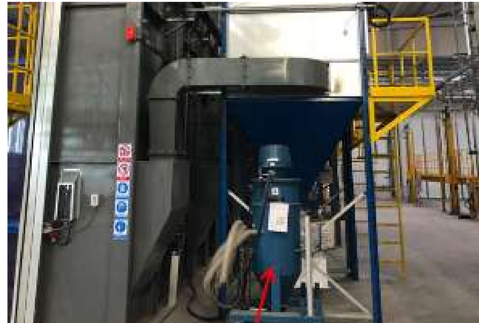
Mobile abrasive resuction installation
