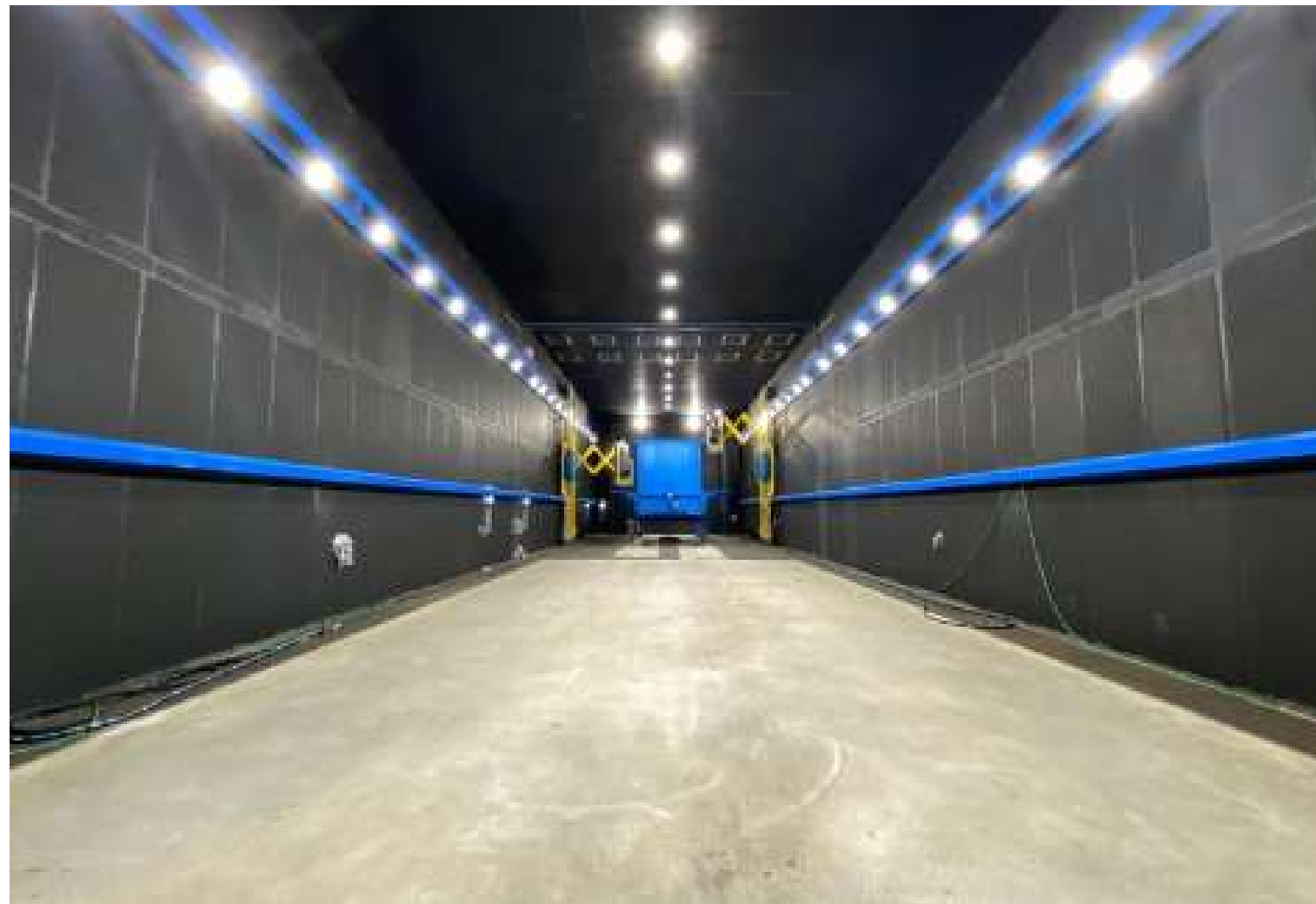
Interior view of a sandblasting room
