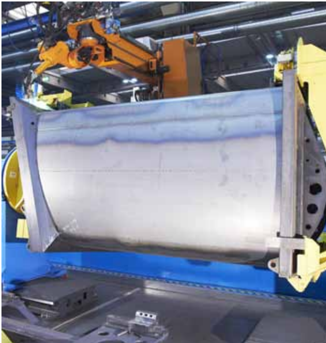
The QRC 350 robot welds the external seam of the container.
