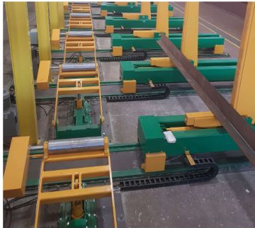
BEAM WELDING / ROTATION
